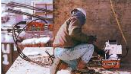
The PE60 used for pre-stressing.
